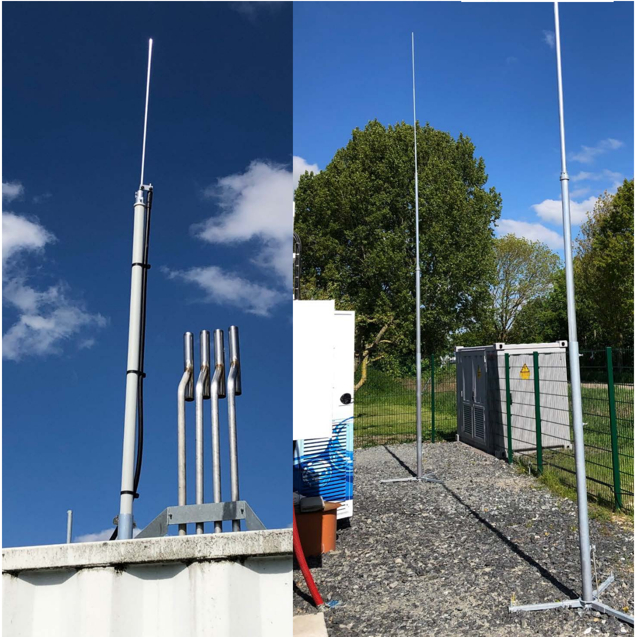
Figure 2: New lightning protection system
