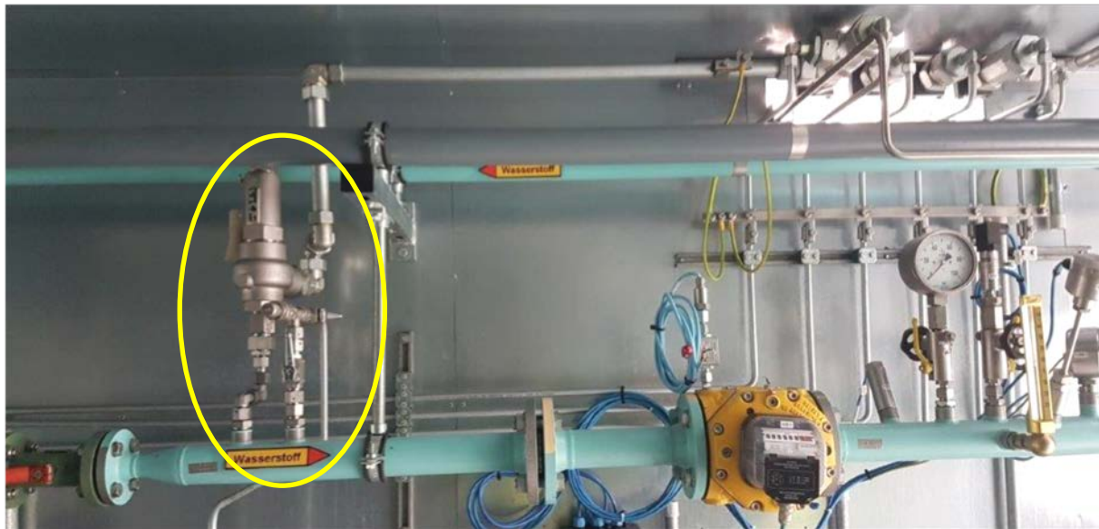
Figure 3: Pressure relief valve (SPV) - setting to 11 bar
